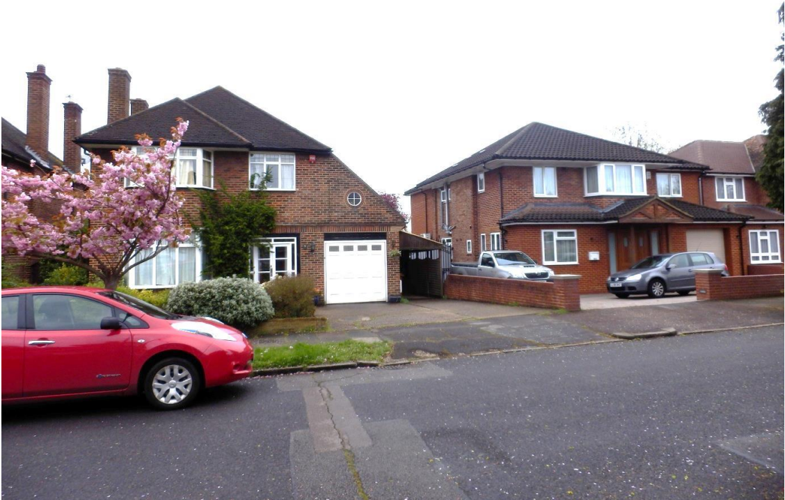
Front of no. 62 (left)
