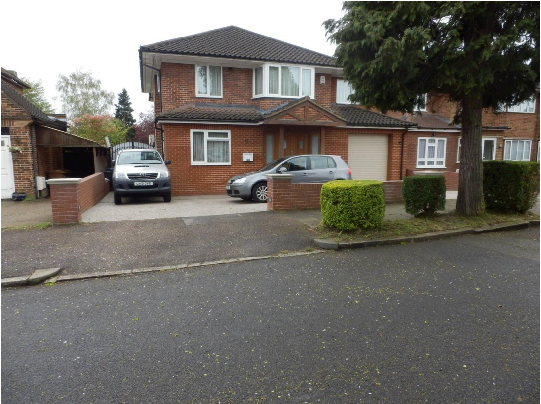
Front of site & access (no. 62 to the left)
